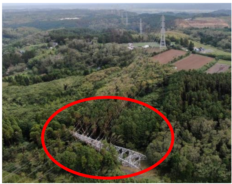
Collapsed transmission tower
