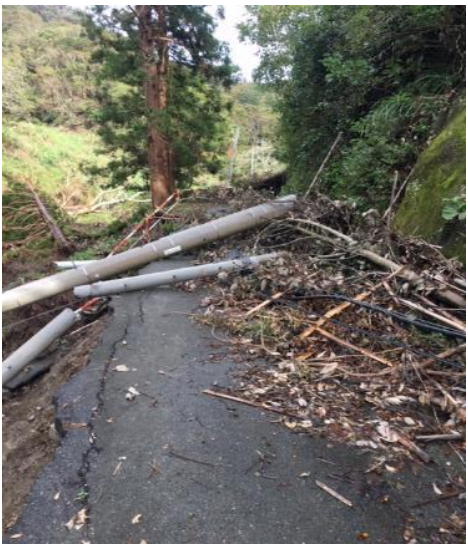
Destroyed utility poles and fallen trees
